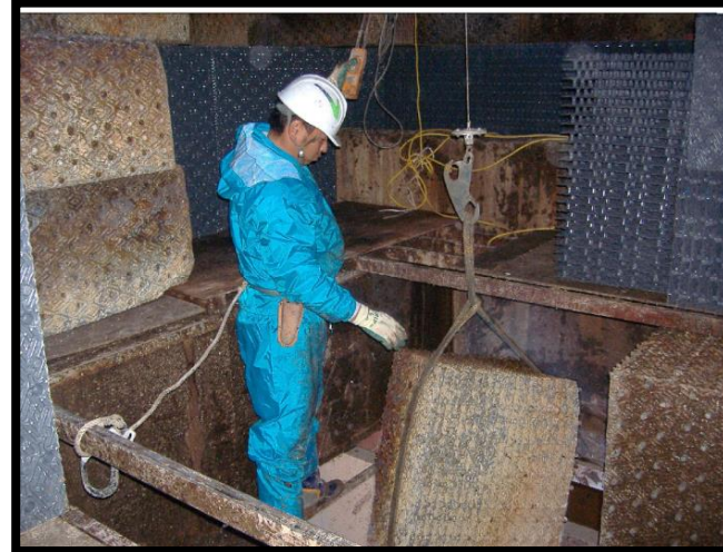
Filling replaced due to buckling by adhering slime and dust gaining the weight
