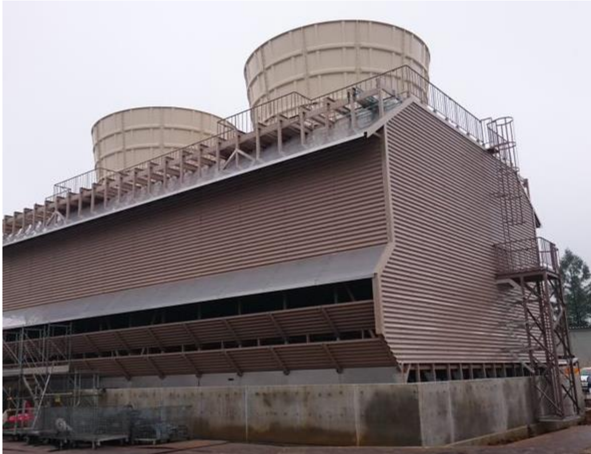
2019 CT for Geothermal Power Plant (Japan) 11,700m 3 /h x 1 units (10 cells)
