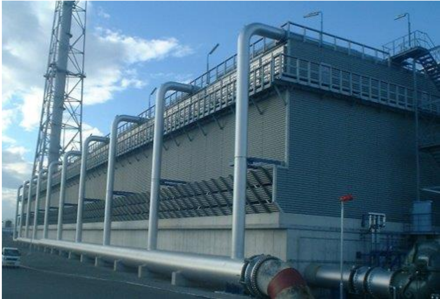
CT for Power Plant (Japan) 30,000m 3 /h x 1 unit (10 cells)
