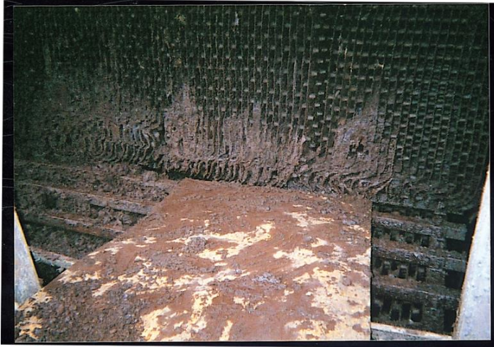
Filling replaced due to low performance by adhering slime and dust
